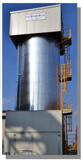
Automatic systems for lime storage pneumatic conveying and injection in electric arc furnace
